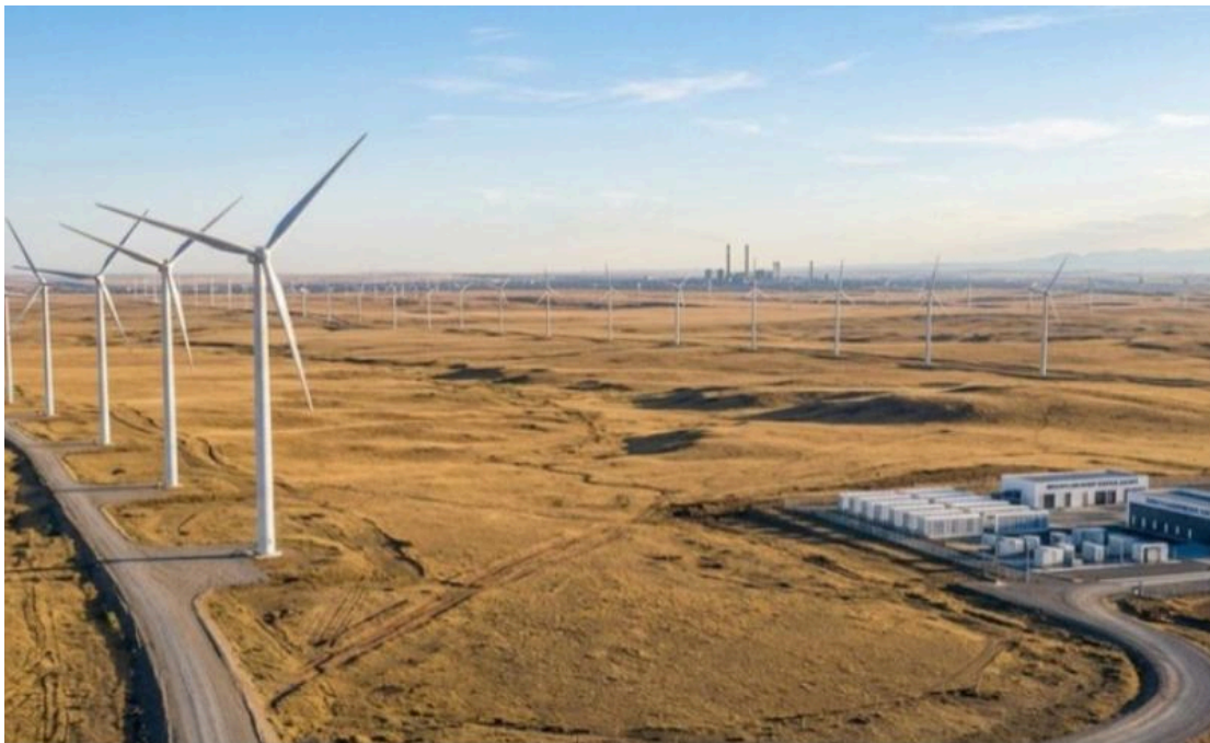
Credit: Ministry of Energy of the Republic of Kazakhstan
